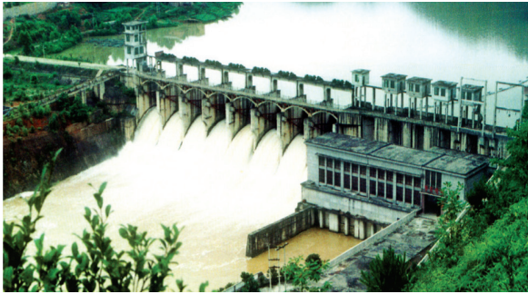
Small hydropower station in Chaling County, Hunan Province
